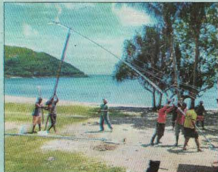
Wind turbines going up to provide power for the water desalinator, lights and refrigeration.
